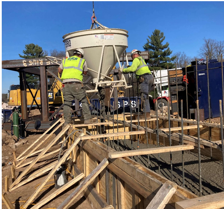
November 1, 2022 - Pouring east abutment footing.
