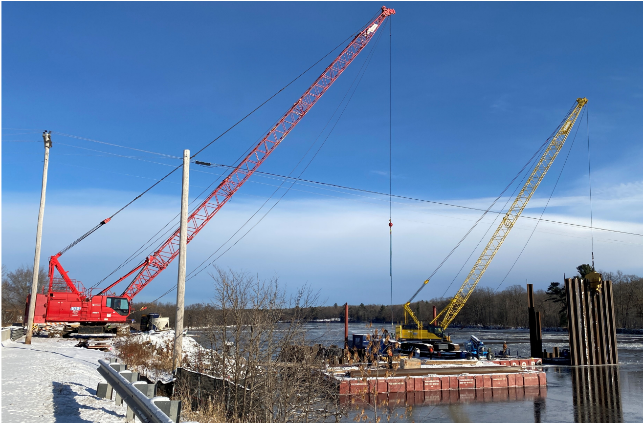
December 1, 2022 - Driving pier 2 cofferdam.
