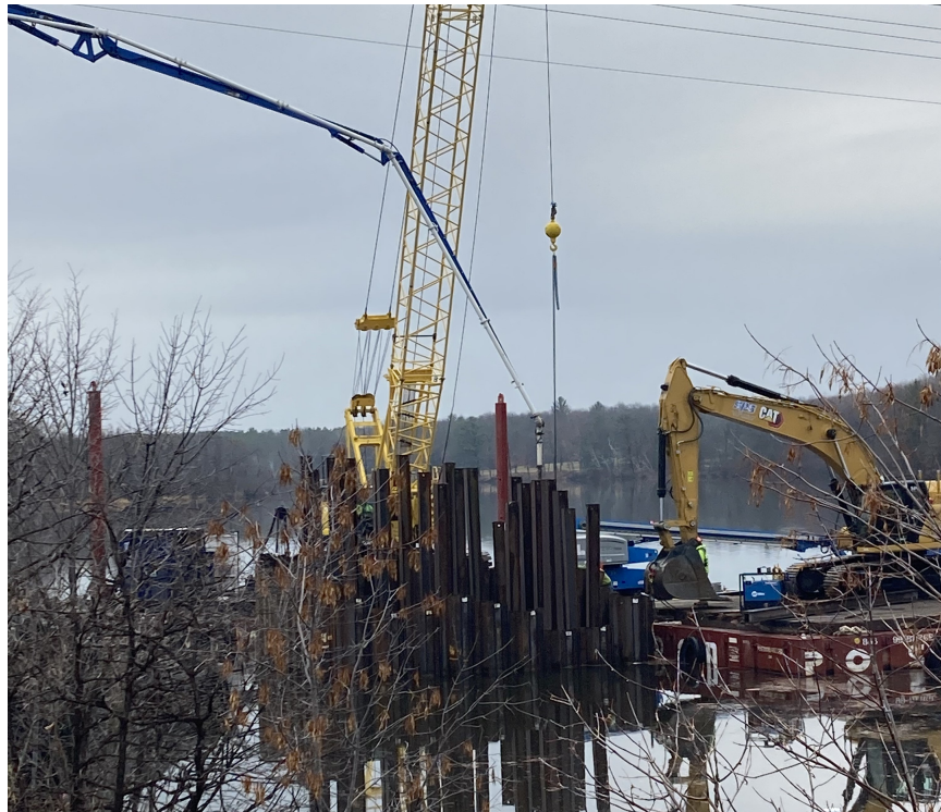
November 9, 2022 - Tremie and pump truck to pour pier 1 cofferdam seal.
