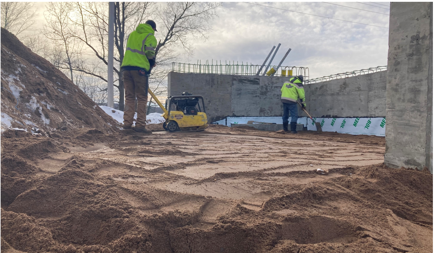
December 6, 2022 - Using a plate compactor and backfilling the east abutment.
