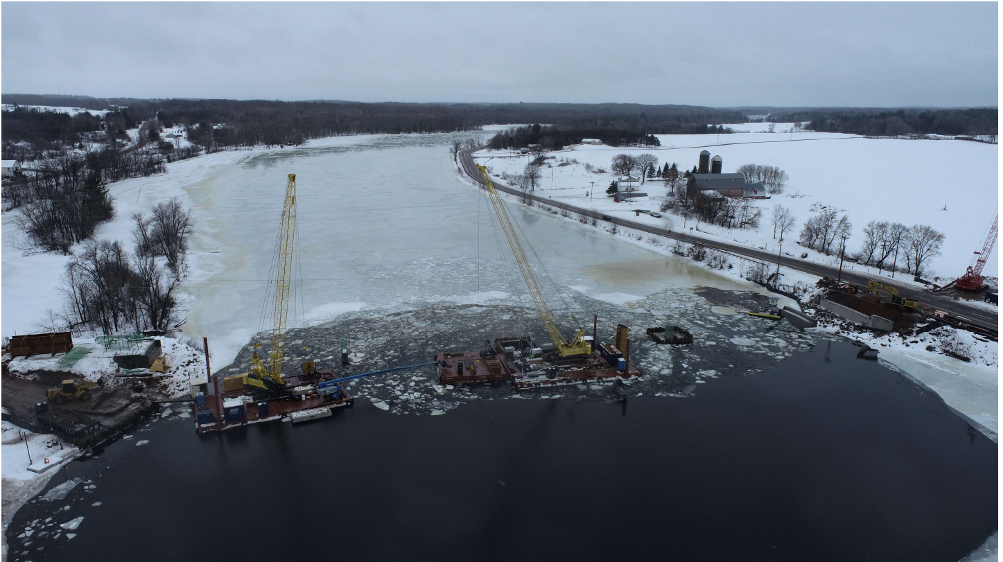
January 17, 2023 – Drone photo of entire bridge length. Both abutments are poured and all 4 piers are in different stages of construction.
