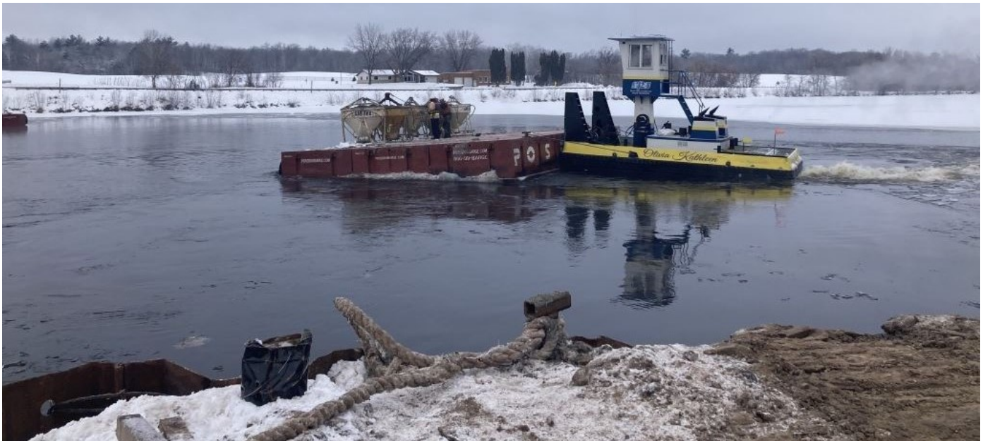
January 6, 2023 – Transporting concrete to pier 2 and pier 3 cofferdam, the concrete trucks deposit the material into 5 crane buckets lined up on a barge. Operator then uses the tugboat to move the barge to pier location. Buckets are lifted with the crane to pour concrete in place.
