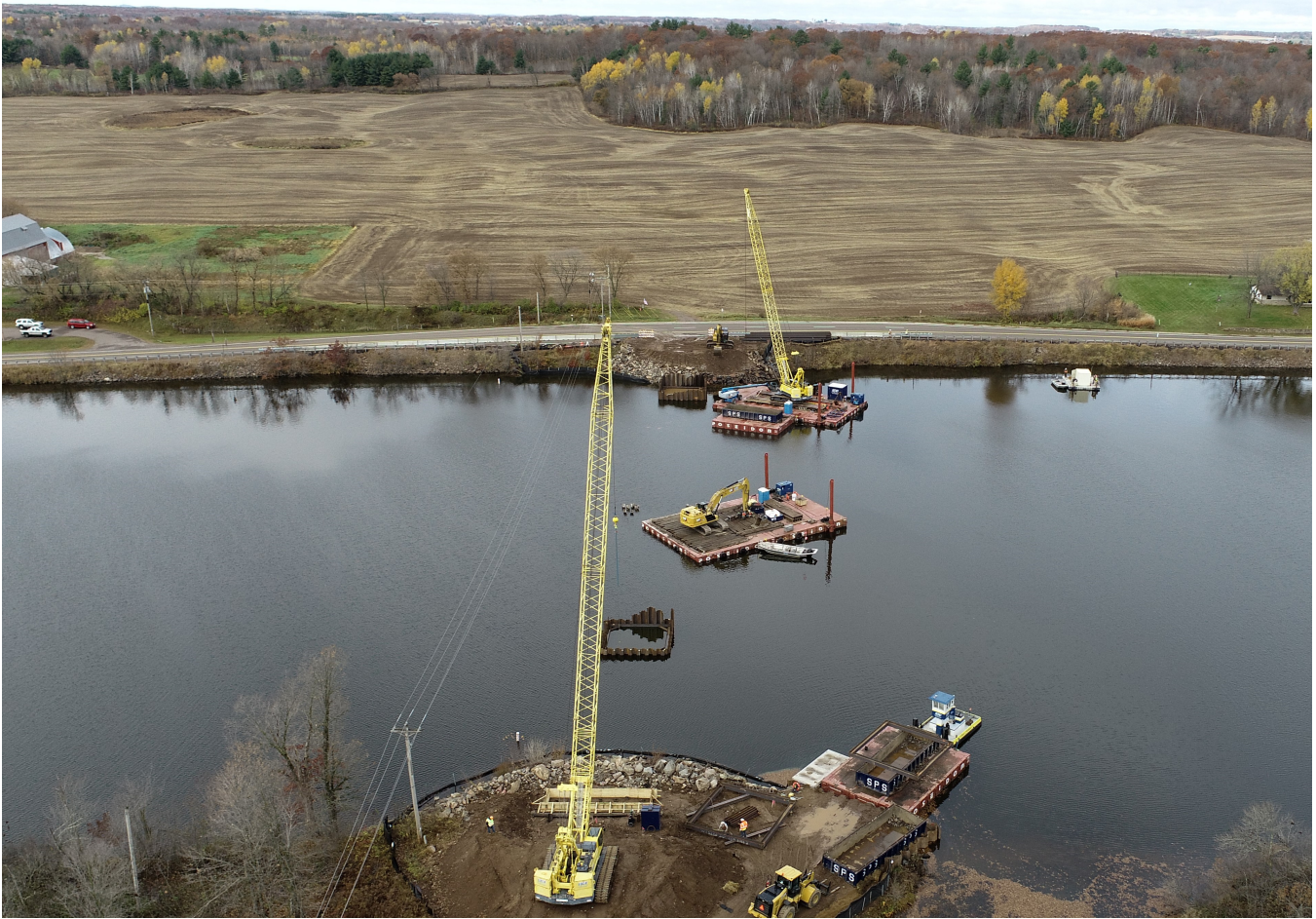
October 25, 2022 - Cofferdams in place for pier 1 and pier 3. Old center pier still in place.
