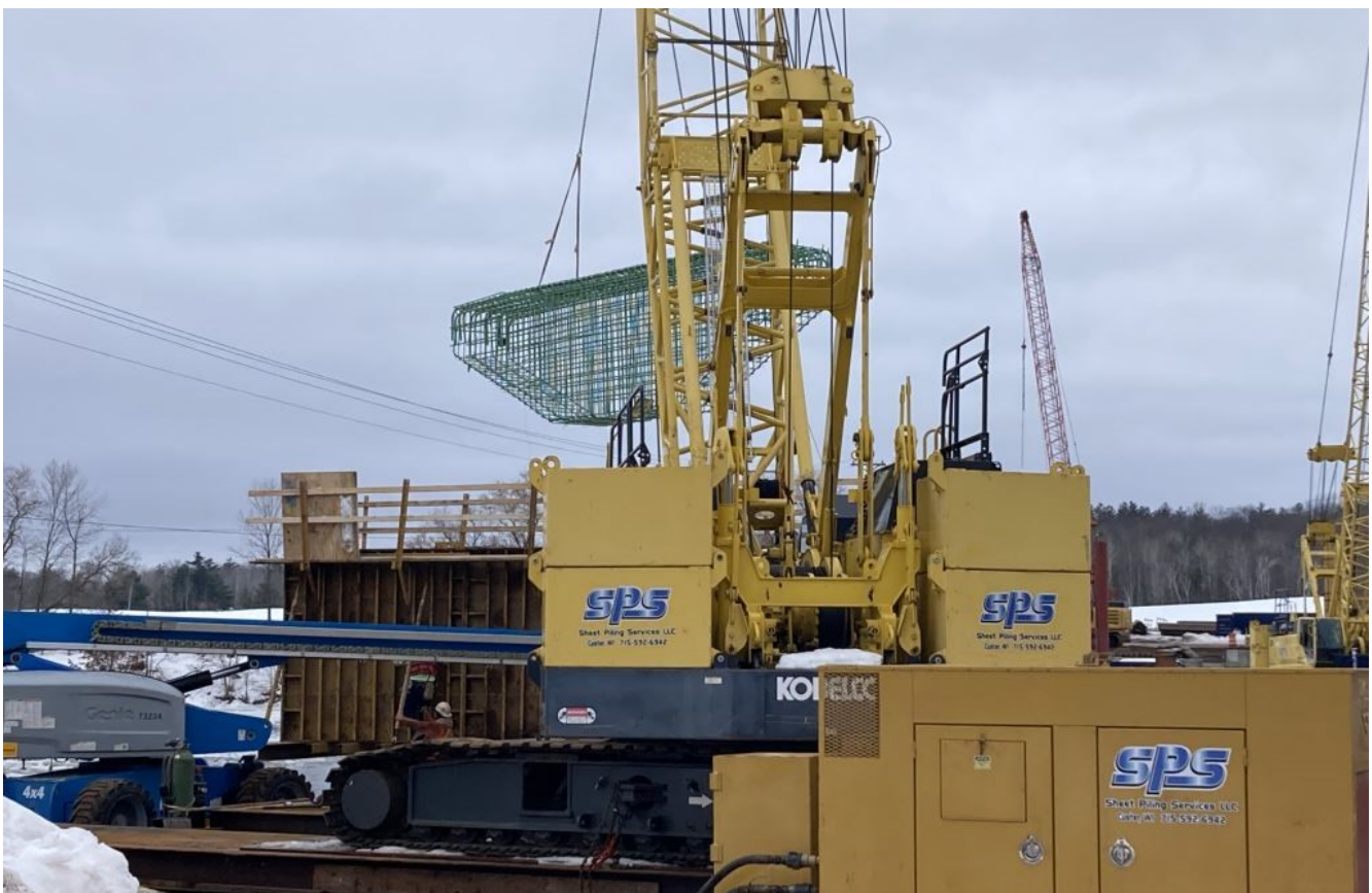
January 18, 2023 – Crane is lifting pier cap 4 rebar cage into place.
