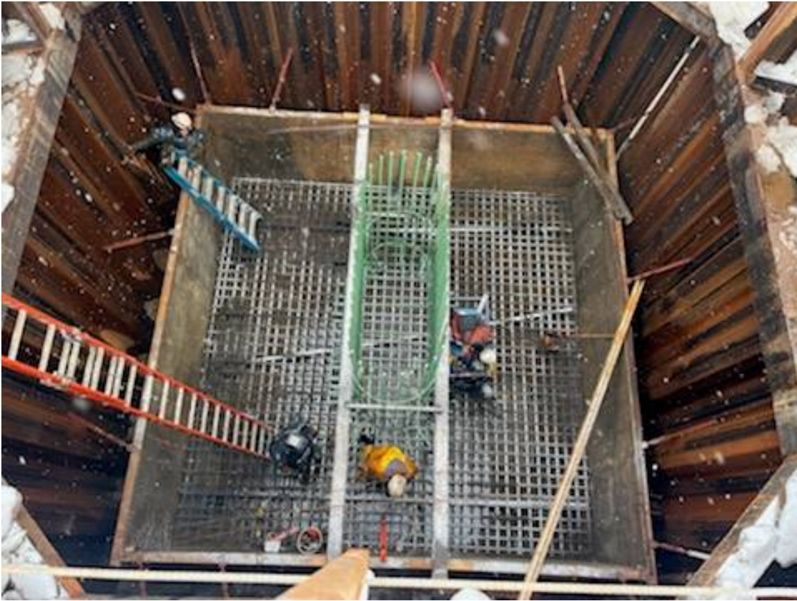
January 5, 2023 – Prepping for pier 2 footing concrete pour. View inside the cofferdam. Rebar cage for stem is visible.
