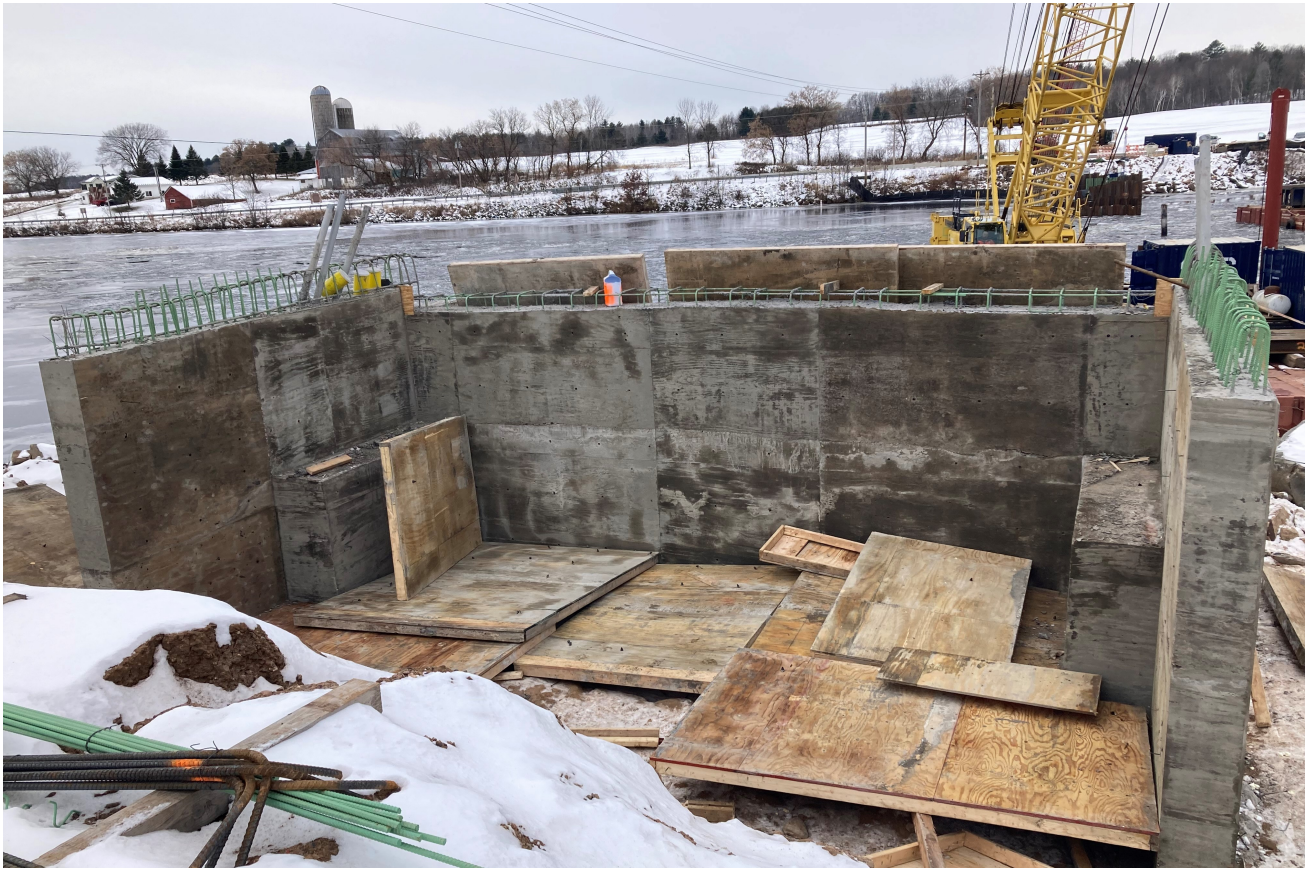
December 5, 2022 - Removing forms from east abutment.
