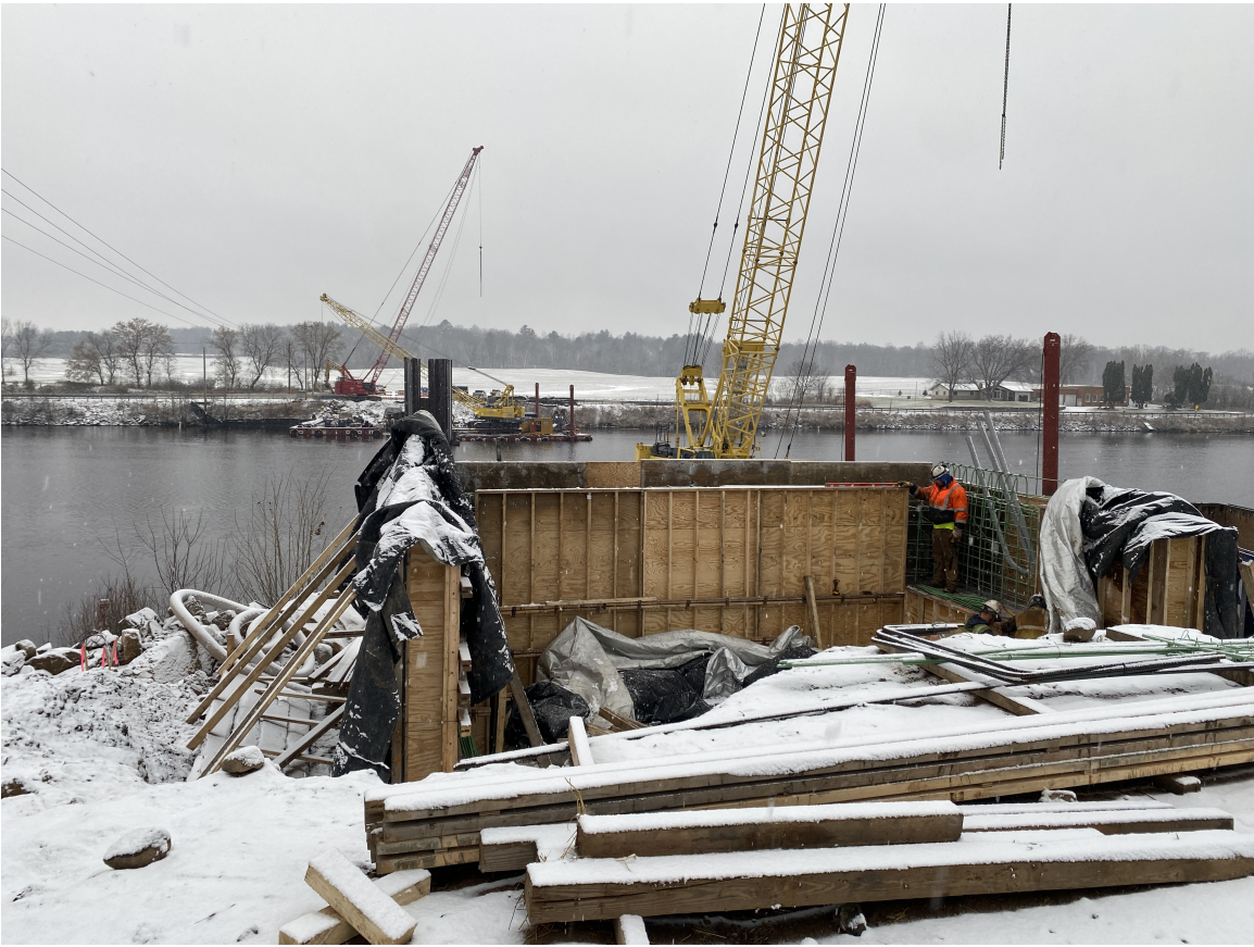
November 29, 2022 - East abutment formed up.
