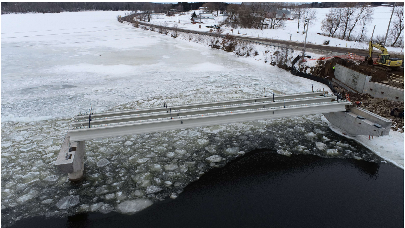
Facing south. Three beams are already set by 10am. This is at the west end of the bridge spanning from pier #1 to pier #2.
