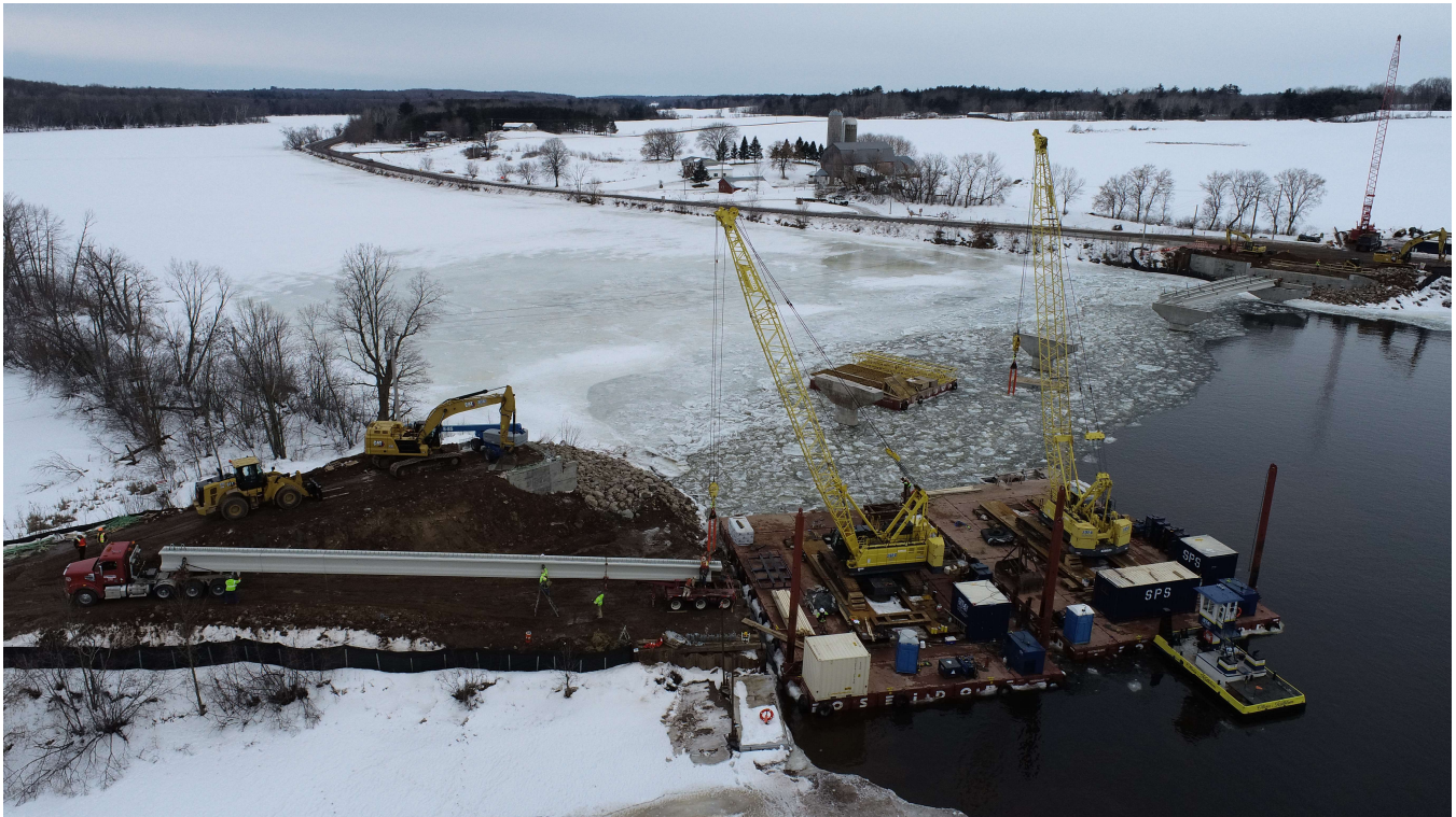
Backing the beam down the access road towards the two cranes.
