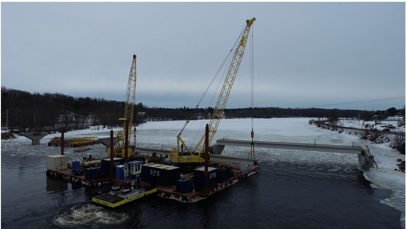
The barges approach the location for setting the beam.
