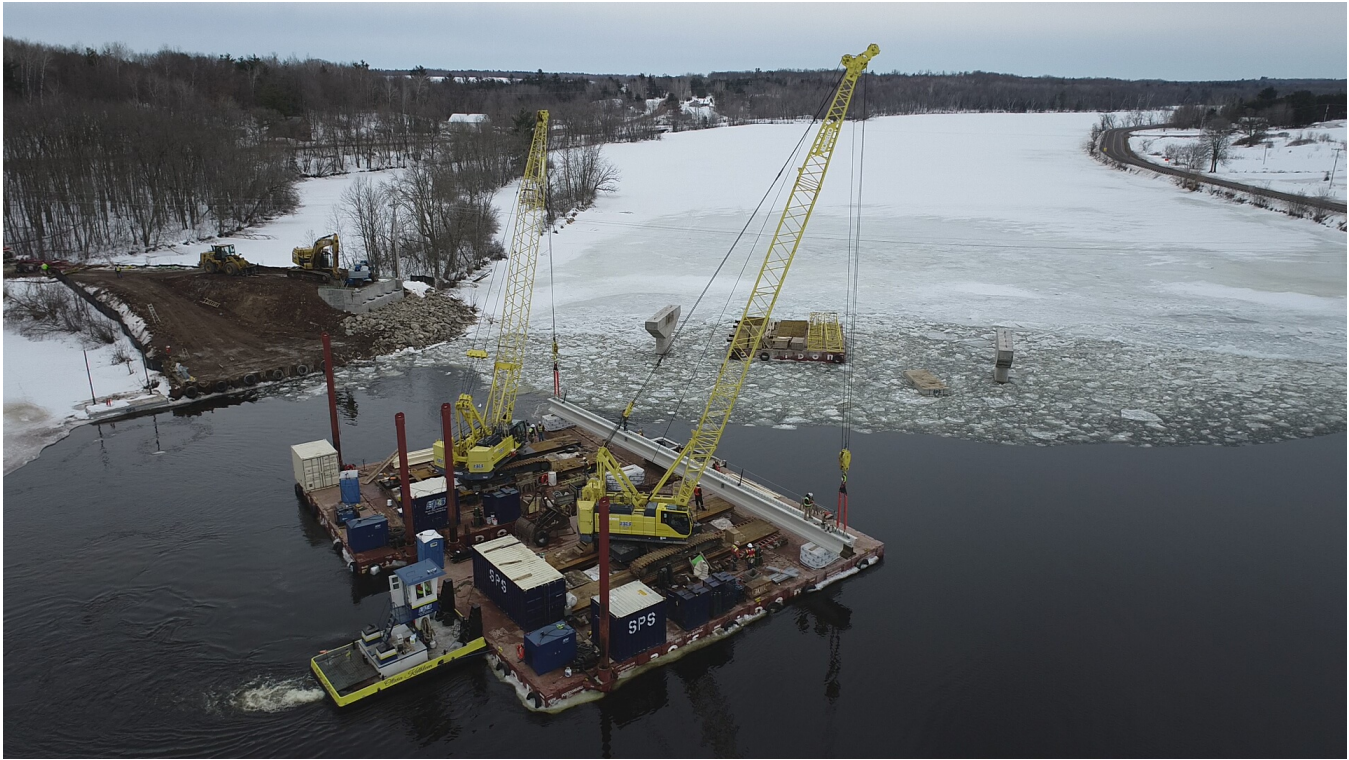
The beam is set on blocks and the tug boat pushes the two barges across the river.
