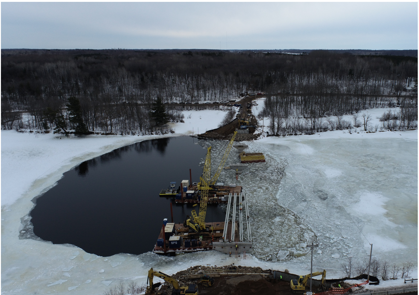
Facing east. 4 of 5 beams have been set.
