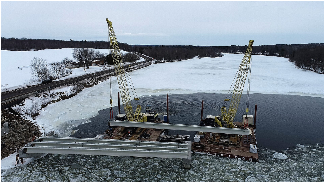
The two cranes lift the beam together and move it into place.
