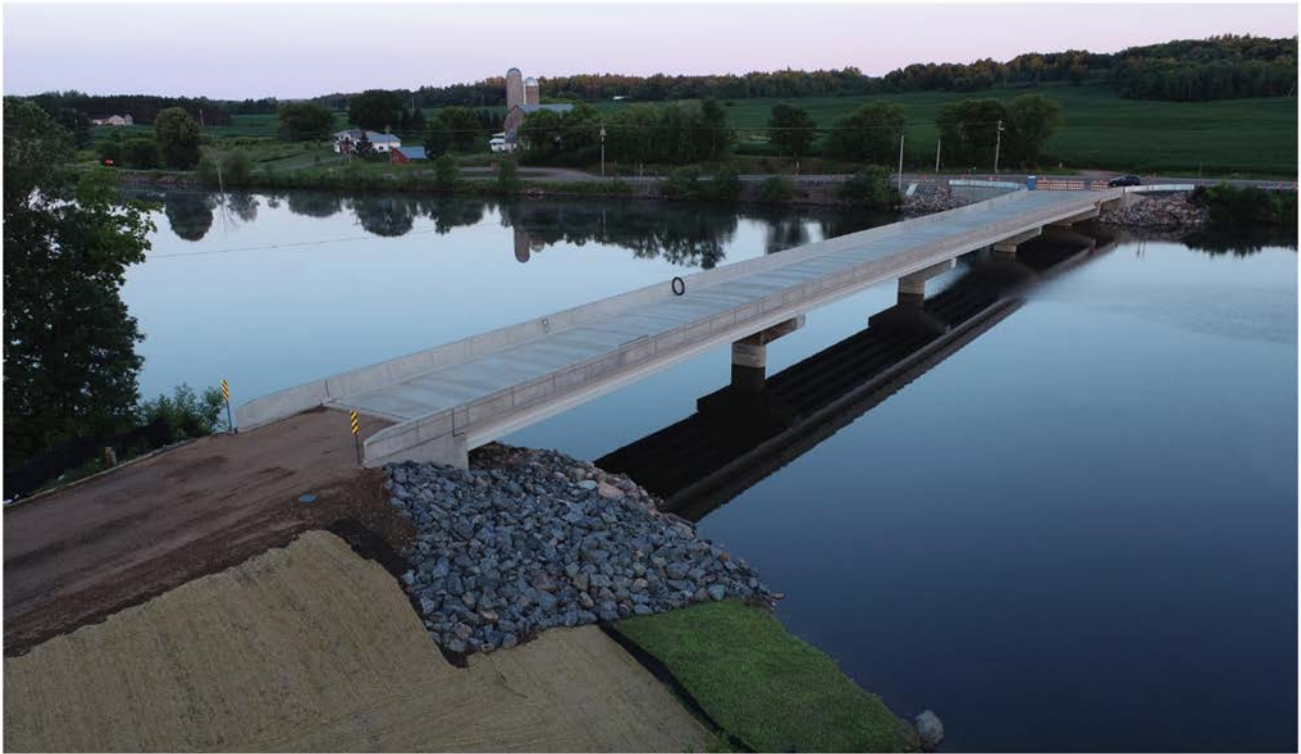
July 11, 2023 – Completed Bridge
