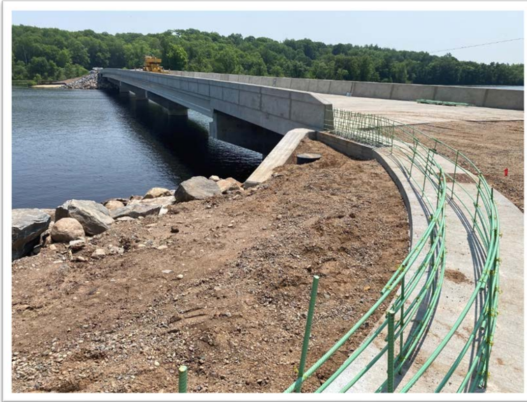
June 22, 2023 – Reinforcement for N/W Barrier Wall
