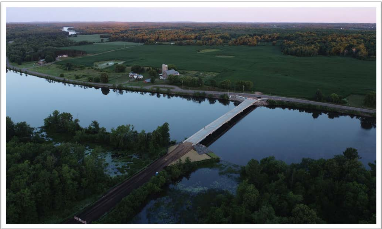
July 11, 2023 – Completed Bridge
