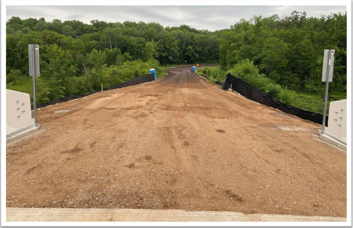
July 13, 2023 – CTH TT Causeway Ready for Pavement
