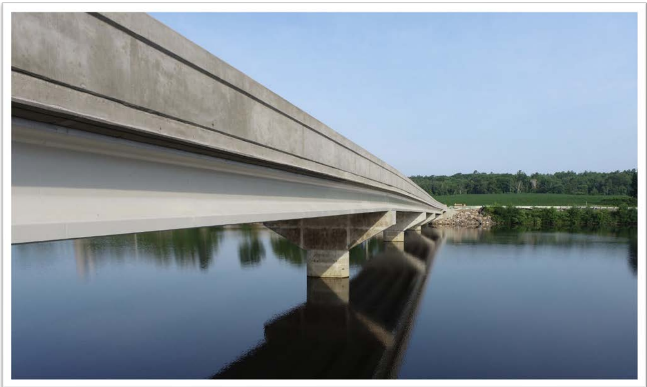
June 23, 2023 – Completed Bridge Side View
