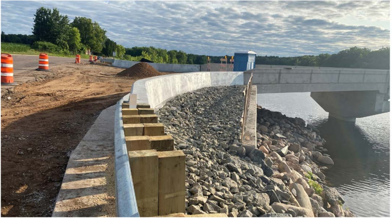
July 6, 2023 – Completed S/W Barrier Wall and Riprap
