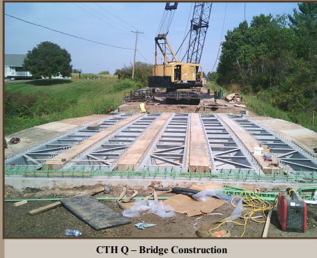
CTH Q – Bridge Construction
