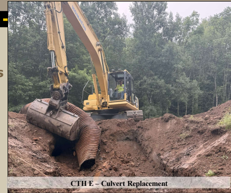
CTHE – Culvert Replacement
