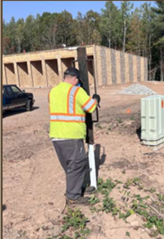
911 Addressing Marker Installation
