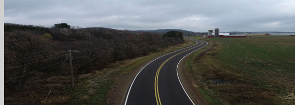
2024 – CTH DD Paving
