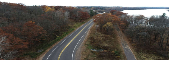
2023 – CTH TT Paving
