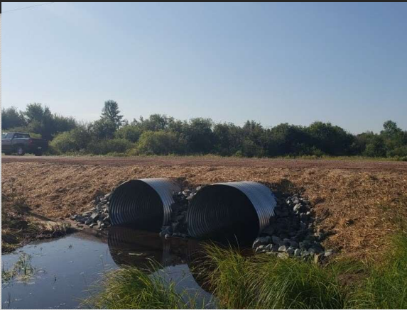
2022 – CTH W Culverts
