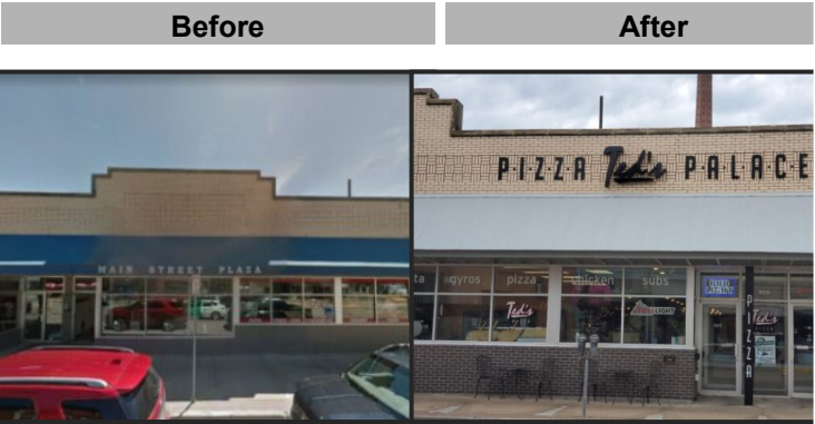
(Below) Ted's Pizza Palace (Dunn County) — Ted's Pizza Palace in Menomonie celebrated its 50th anniversary in 2020. Owners Jim and Kim Gounakis simultaneously perform renovations to their building. A Façade Loan assisted with the pictured exterior renovations.
