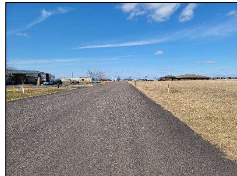
Lakeland Drive Looking North
