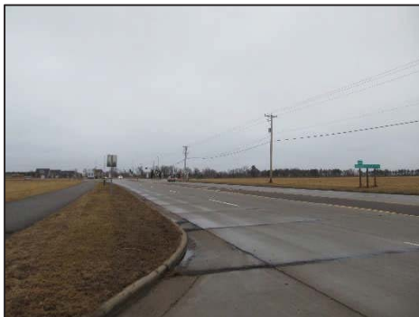
CTH I Looking Easterly
