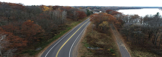
2023 – CTH TT Paving
