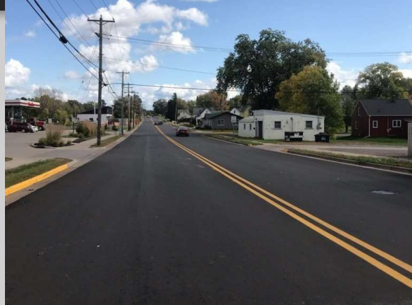
2023 – CTH X in Stanley Paving
