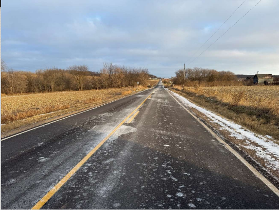
2024 – CTH HH Paving
